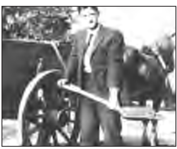
T.F. Gullixson, PhD, turning the first shovel of dirt where Trinity Hospital now stands. The photographer was Otto Ellison, a well-known businessman and longtime member of the Board of Trustees.
